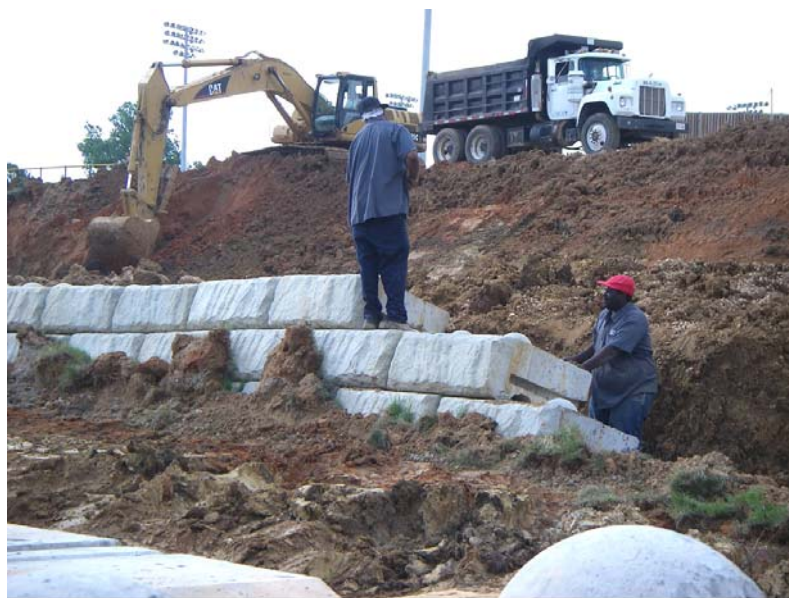
Figure 4. Excavation of slump block and removal of the tilted retaining wall. Each concrete block in the wall weighs 2,000 pounds and is fastened by dome and socket joints. Removed blocks are stacked in the foreground for reassembly later. Picture (digital CD #42) taken June 4, 2008.
