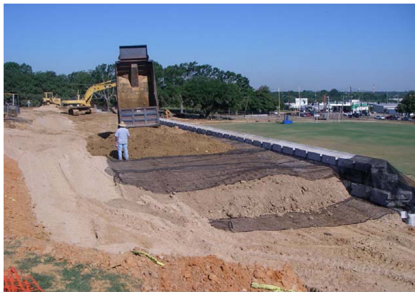
Figure 6. Layers of geogrid fabric and soil are placed behind the upper retaining wall at Millsaps College. The geogrid fabric ties the layers into a coherent block that resists the fractures and shearing responsible for slope failures. Picture (digital CD #47) taken on July 2, 2008.
