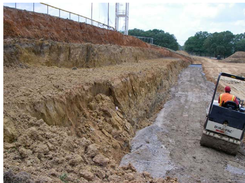
Figure 1. Excavation for a new football field at Millsaps College in Jackson, Mississippi. The lower two tiers in the foreground consist of weathered Yazoo Clay. The upper tier is terrace sand, which drapes over the Yazoo Clay of the bottom tiers in the distant hillside. The crushed limestone floor is the foundation for a retaining wall. Extra stone is placed at the base of a small slump in the foreground. Picture (digital CD #41) taken on May 23, 2007.
