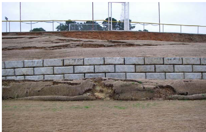
Figure 2. Slump in Yazoo Clay pushed the retaining wall up and out as seen from the new football field at Millsaps College in Jackson, Mississippi. The slump scarp cuts near the observation tower of the upper field, and the toe is elevated in front of the retaining wall like a roll of carpet. Picture (digital CD #42) taken on January 31, 2008.
