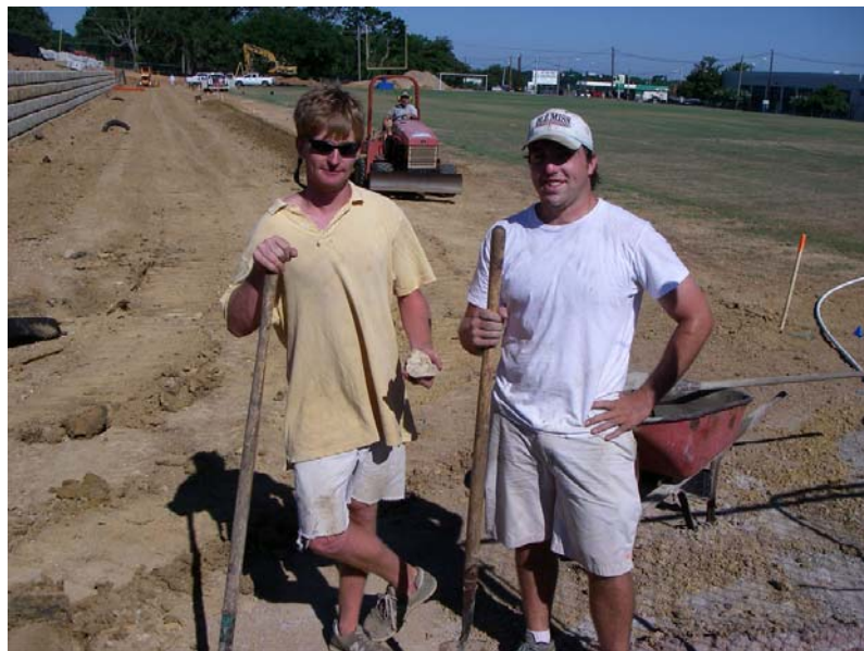
Figure 8. James Bridgforth, holding fossil oyster excavated from irrigation trench, Jared Meyers (right), and Rob Anders on trenching tractor, all with Lakeland Irrigation. James reported, "I'm doing the same thing I did last year." The main line of the first system was taken out by the slump. Picture (digital CD #47) taken on July 1, 2008.
