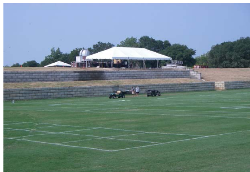
Figure 7. New retaining wall at Millsaps College completed in time for the Saints' summer football camp. The upper wall was extended from 205 to 300 feet to the east (left) of the stairs. Picture (digital, CD #55) taken on July 22, 2008.
