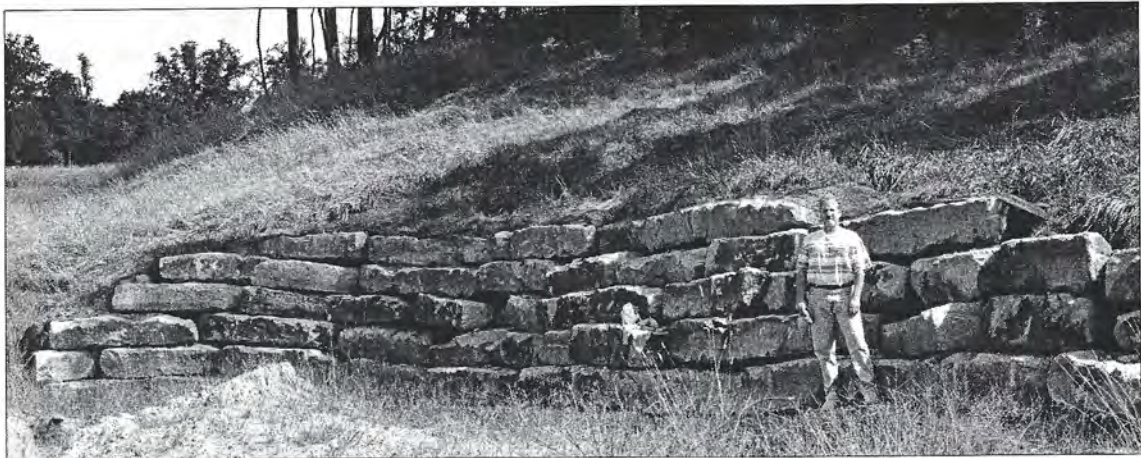
Figure 4 – David Thompson at Tallahatta Sandstone Retainment Wall
