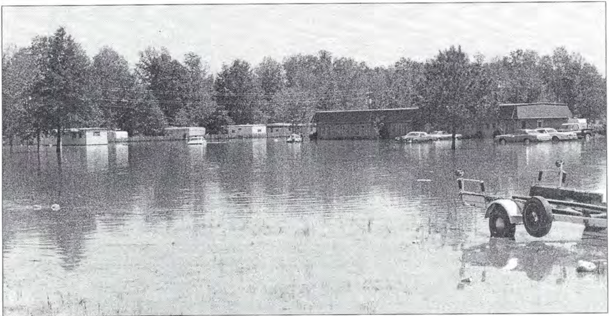
April 15 - Mobile homes below the dam are flooded.
