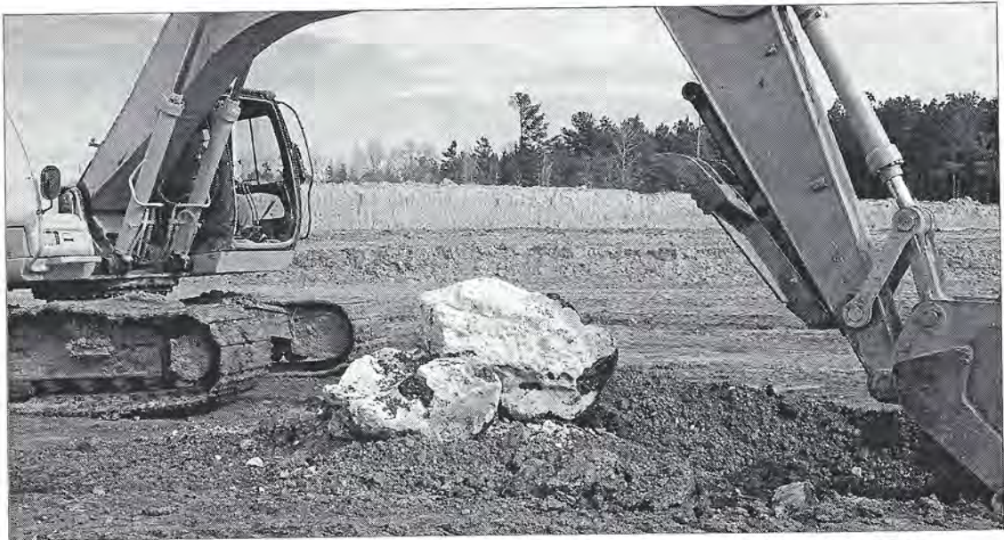
Glendon Limestone boulder excavated from residual clay at the new Brandon High School .
