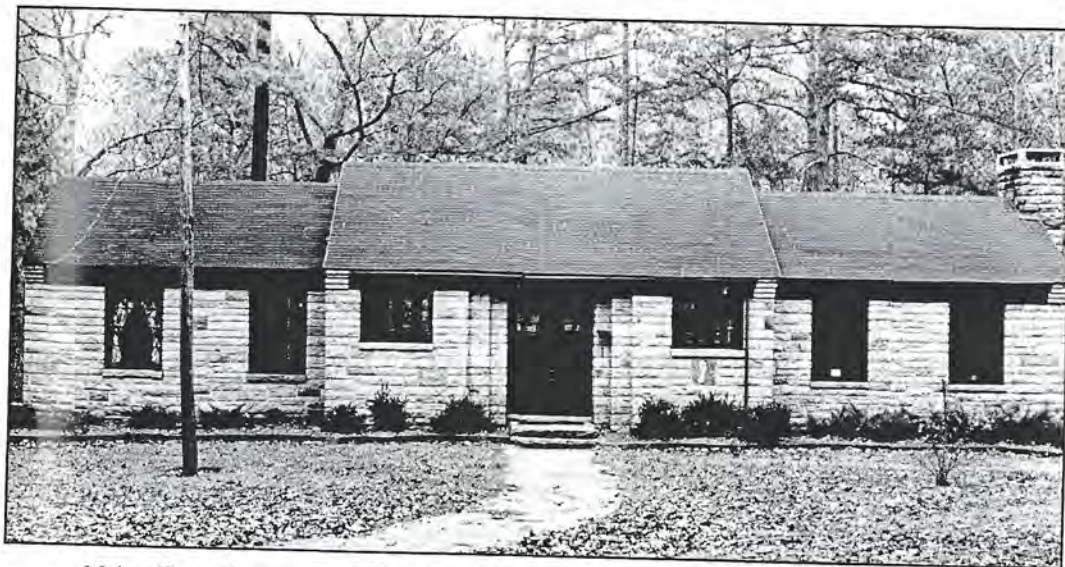
Main office and museum at Tishomingo State Park constructed from the Hartselle sandstone.
