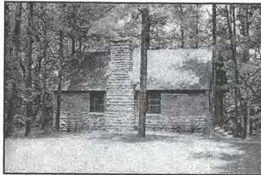
Cabin constructed of Hartselle Sandstone in Tishomingo State Park, Tishomingo Co., MS. Photo by W. S. Parks, June, 1959.
