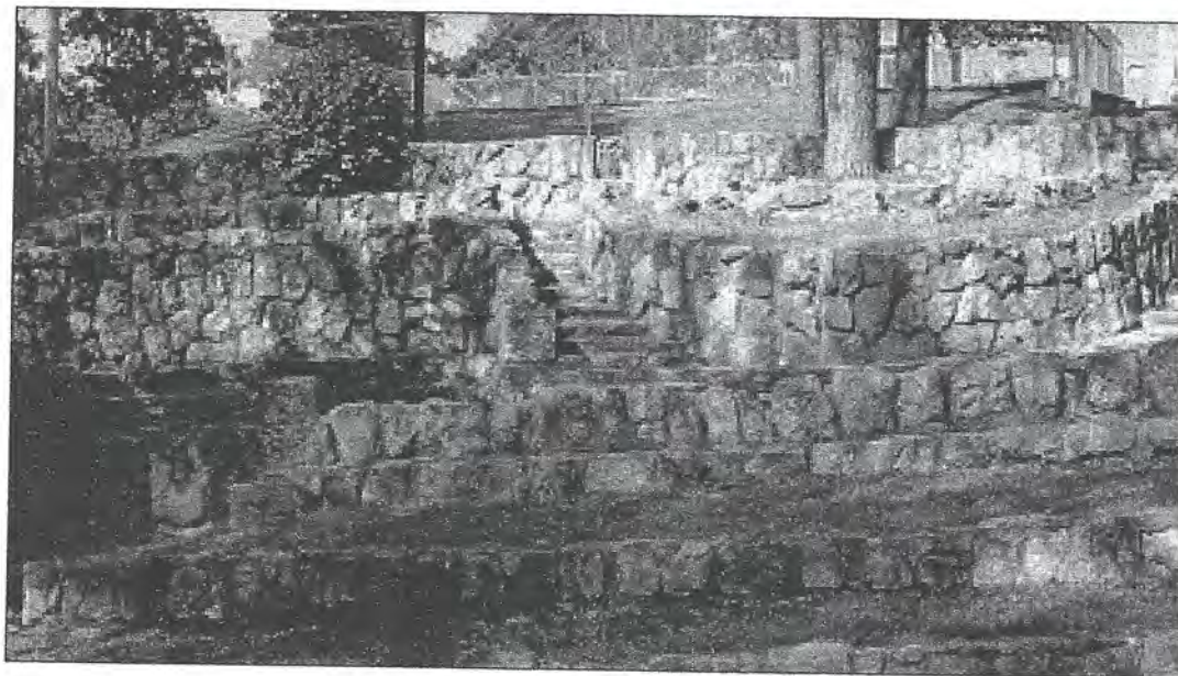
Catahoula stonework at Piney Woods School.
