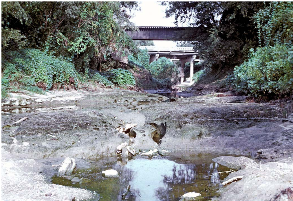
Figure 3. The Moodys Branch formation exposed at Town Creek in Jackson, Mississippi, (MGS locality 1) before the construction of a sewer line across the site. A railroad bridge and the South State Street bridge appear in the background. Picture (Kodachrome slide 155-5) taken in September of 1970.
