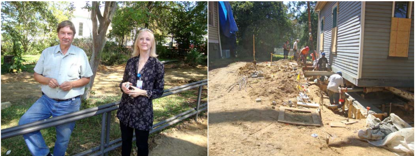
Figure 3. Left, site engineer Britt Maxwell and Manship House Museum director Marilyn Jones. Right, the Manship House rests on steel I beams as a new perimeter skirt foundation is poured by a trailer-mounted boom cement pump. Pictures were taken on October 5, 2012.
