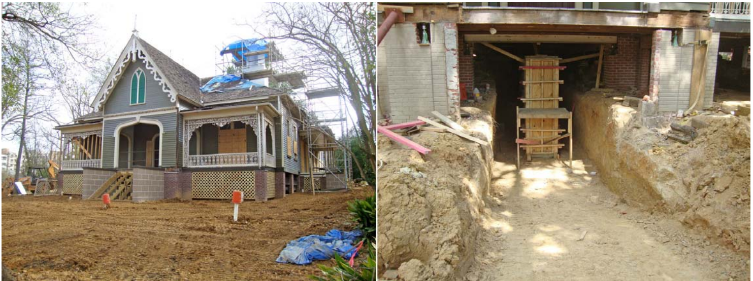
Figure 1. Left, Manship House with new foundation and reconstructed chimneys. Right, construction of new piling at front of house. Pictures were taken on January 29, 2013, on left and August 2, 2012, on right.
