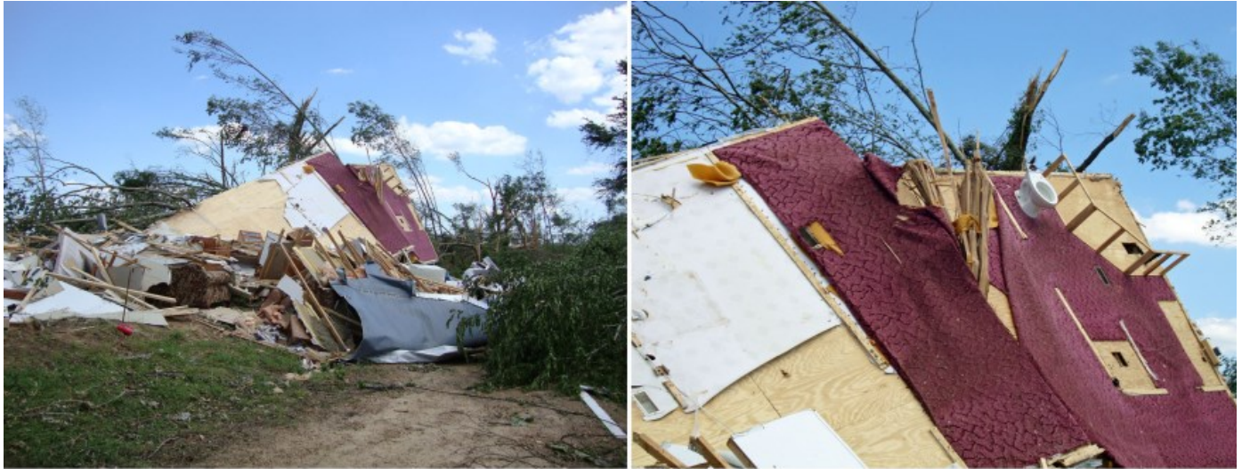
Figure 5. The floor of a mobile home with a very clean toilet west of Highway 49 in Yazoo City impaled on the splintered trunk of a tree. Pictures were taken on April 25, 2010.
